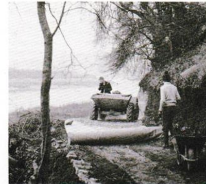
2. Stone laid on filter fabric on new path.
