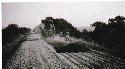
1. Tipping Limestone dust onto remaining ballast
