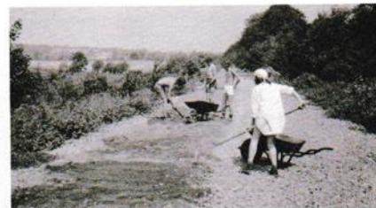
2. Spreading dust and raking level
