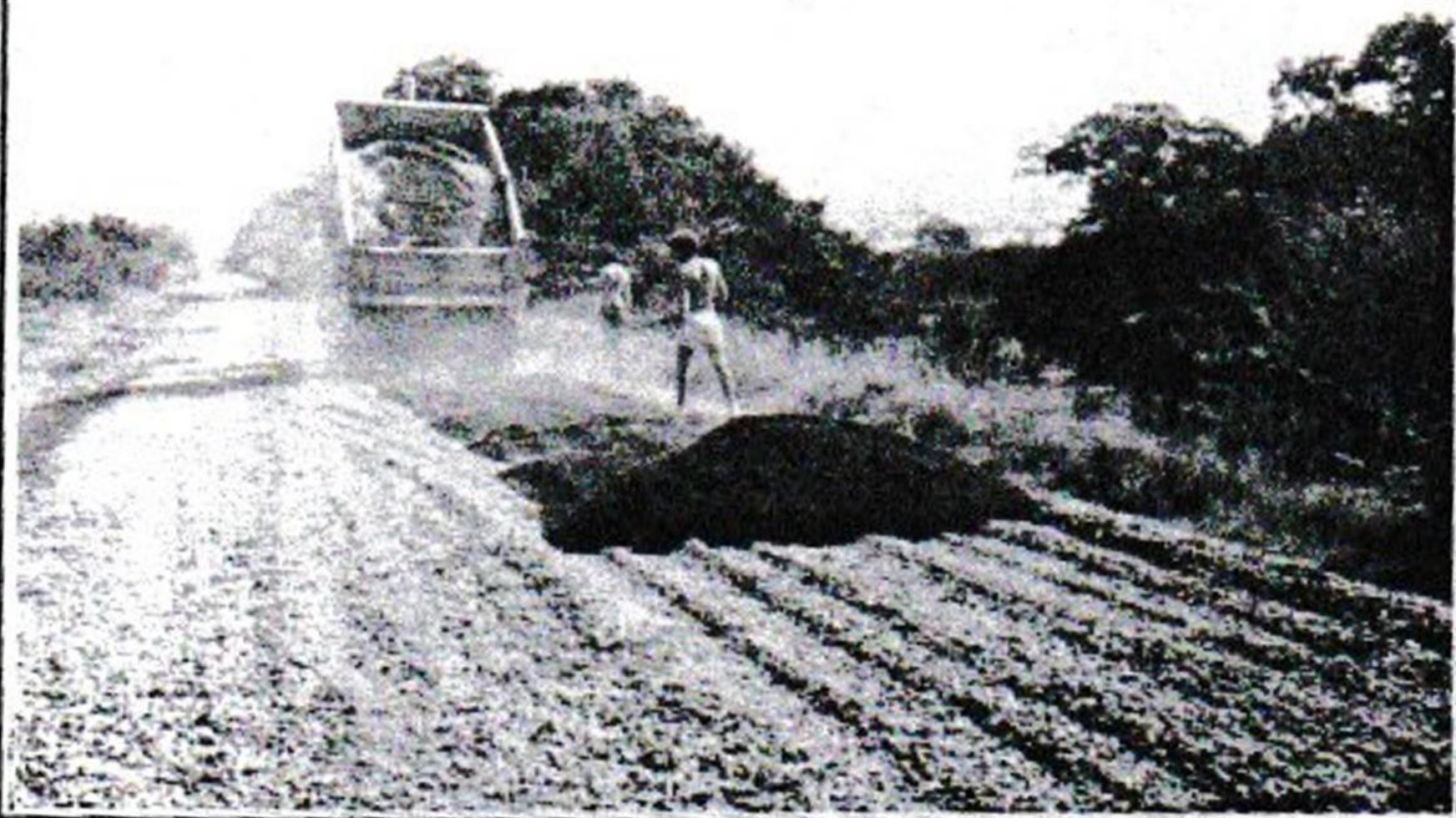
Tipping limestone dust near Bitton.
