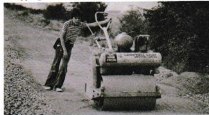
3. Compacting with twin drum vibrating roller
