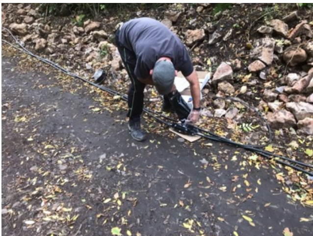
Resin poured into every junction box.
