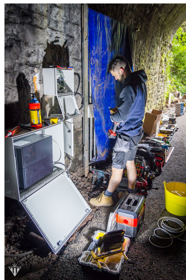
Lights control box in tunnel
