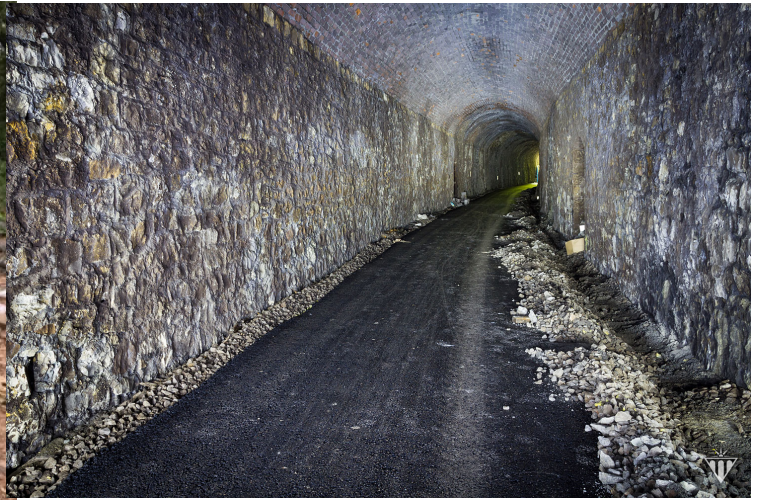
Trench for cables excavated in tunnel
