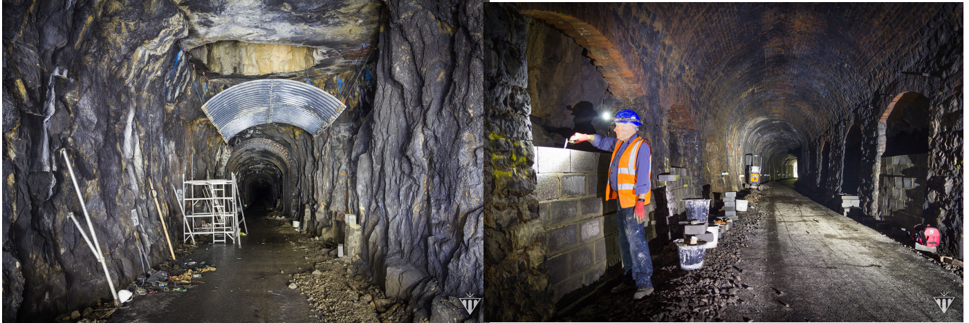
Air shaft shield erected, hung on chains.
