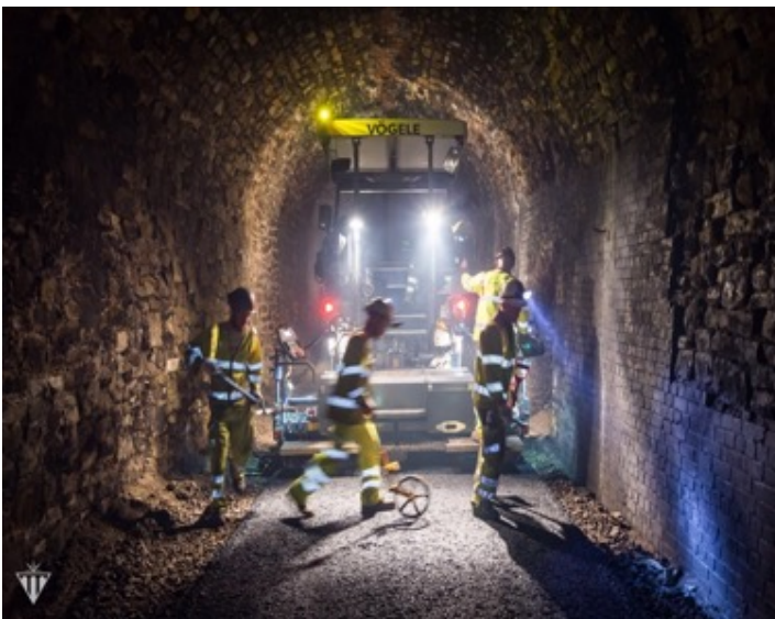
Blacktop being laid in tunnel.
