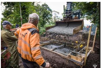
By Monday morning the first shuttering and reinforcement were in place and the concrete base of the West abutment was poured, without a hitch.
