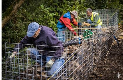
The gabion team found time to reinforce the approach ramp above the large culvert too.
