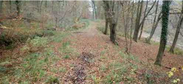
NW6 The existing forest track above the railway through Norchard Wood. This has a sound shape but would need a new stone surface
