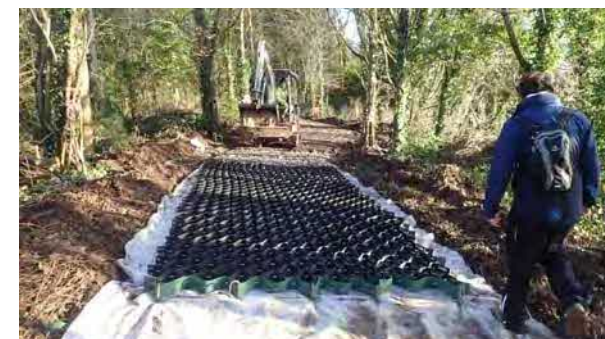
Picture showing construction through woodlands using “tree cell”: view of completed path below. Ashton Park Estate, Bristol, February 2020
