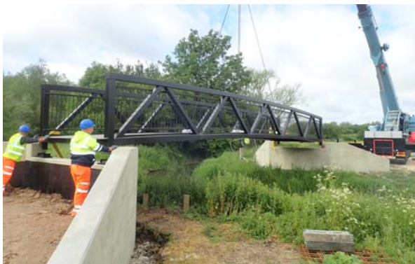
Picture of Haydon Hill Bridge being lifted into place
