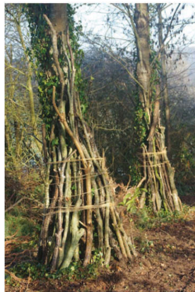
View of tree protection fascines used on adjacent trees in Ashton Court – Listed Repton Estate.
