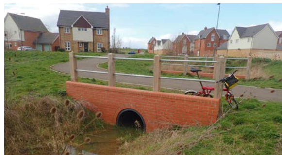
View of existing culverts and brick head walls in the flood plain
