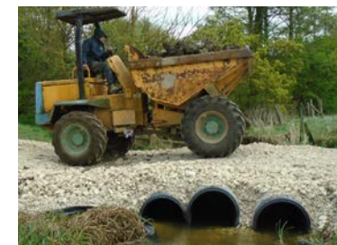
View of temporary 'Irish' bridge works crossing used at Fleet Marston
