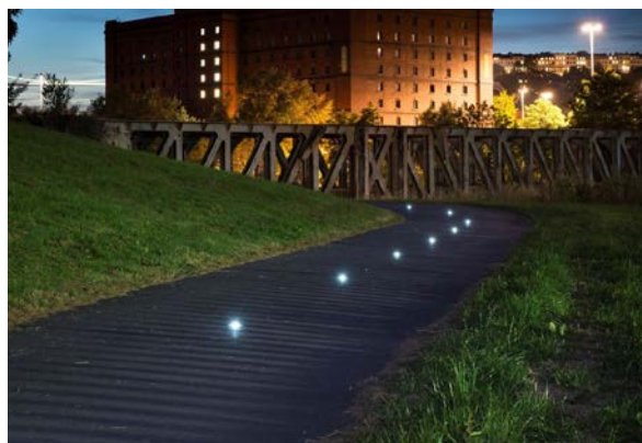
Example of recessed LED greenway lighting (Bristol)
