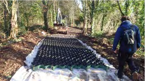
Picture showing construction through woodlands using "tree cell": view of completed path below. Ashton Park Estate, Bristol, February 2020
