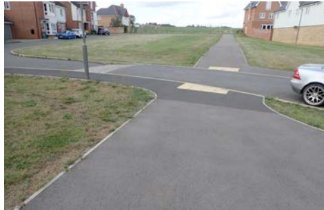
View of existing Avalon Street raised road crossing
