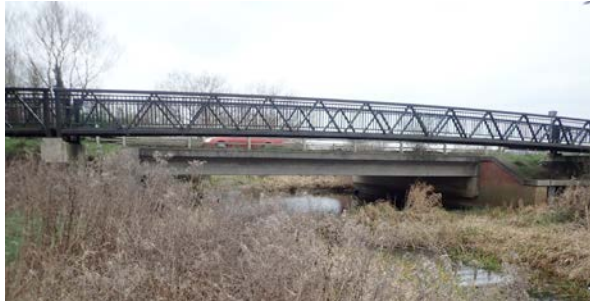
View of similar truss bridge adjacent to Bicester Road. The planned bridge will be 2.5m wide.
