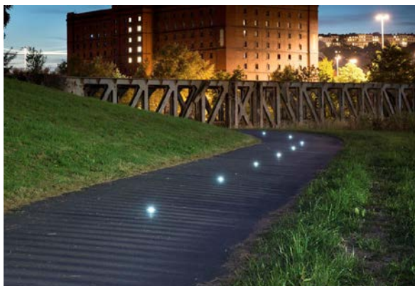
Example of recessed LED greenway lighting (Bristol)
