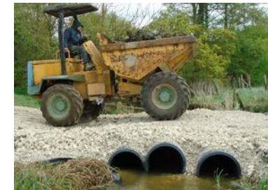
View of temporary 'Irish' bridge works crossing used at Fleet Marston
