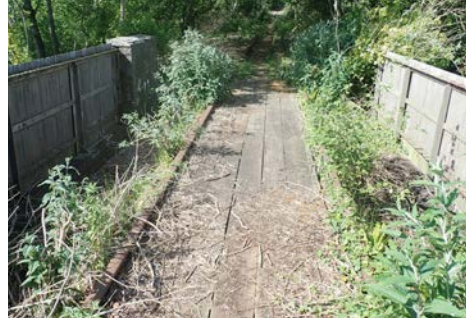
View of bridge at present showing the remaining continuously welded rails and timber decking
